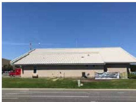
Standing Seam Metal Roof on the Fire Station 72 Richland, WA (pictured above)
