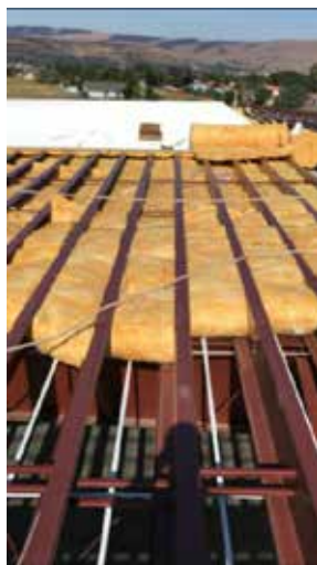
Standing Seam Metal Roof over R-38 batten insulation on a pre-engineered building (middle of page)
