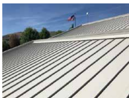
Standing Seam Metal Roof on the Fire Station 72 Richland, WA (pictured above)
