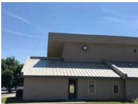
Standing Seam Metal Roof on the Fire Station 72 Richland, WA (pictured above)
