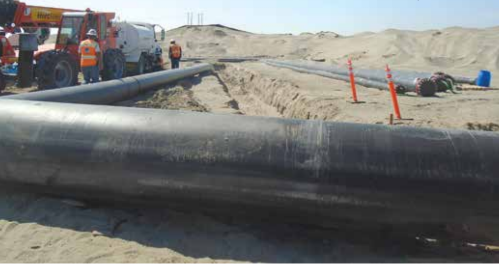
Trenching and installation of water utility pipe. Photo courtesy of Burnham.
